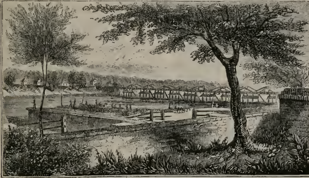
VIEW FROM THE SITE OF FORT CORNWALLIS. 2
